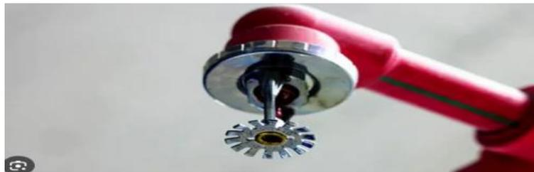
Gambar 2. 6. Alat *Sprinkler* Pemadam Api (Sumber Bromindo)
