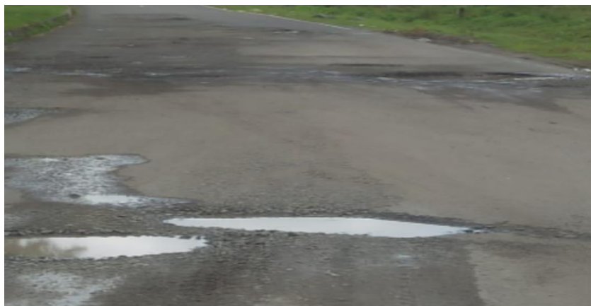
Gambar 2. 6 Lubang ( Potholes )
